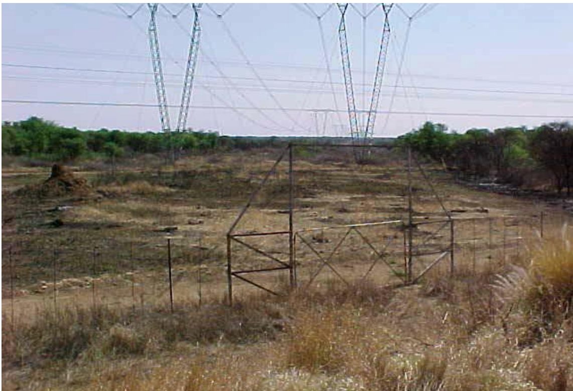
Figure 4: A game fence as used on the Matimba-Spitskop 1&2 lines. Note that the top section has been omitted as per the latest 5m game gate design
