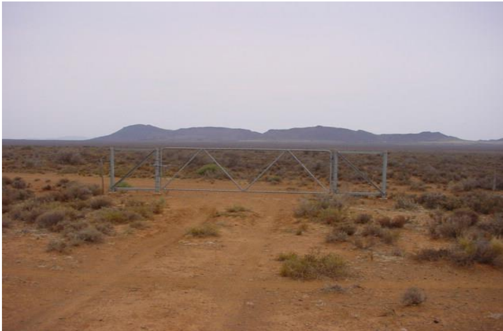
Figure 3: Standard Eskom gate as was used on the Hydra- Droërivier No 3 Line
